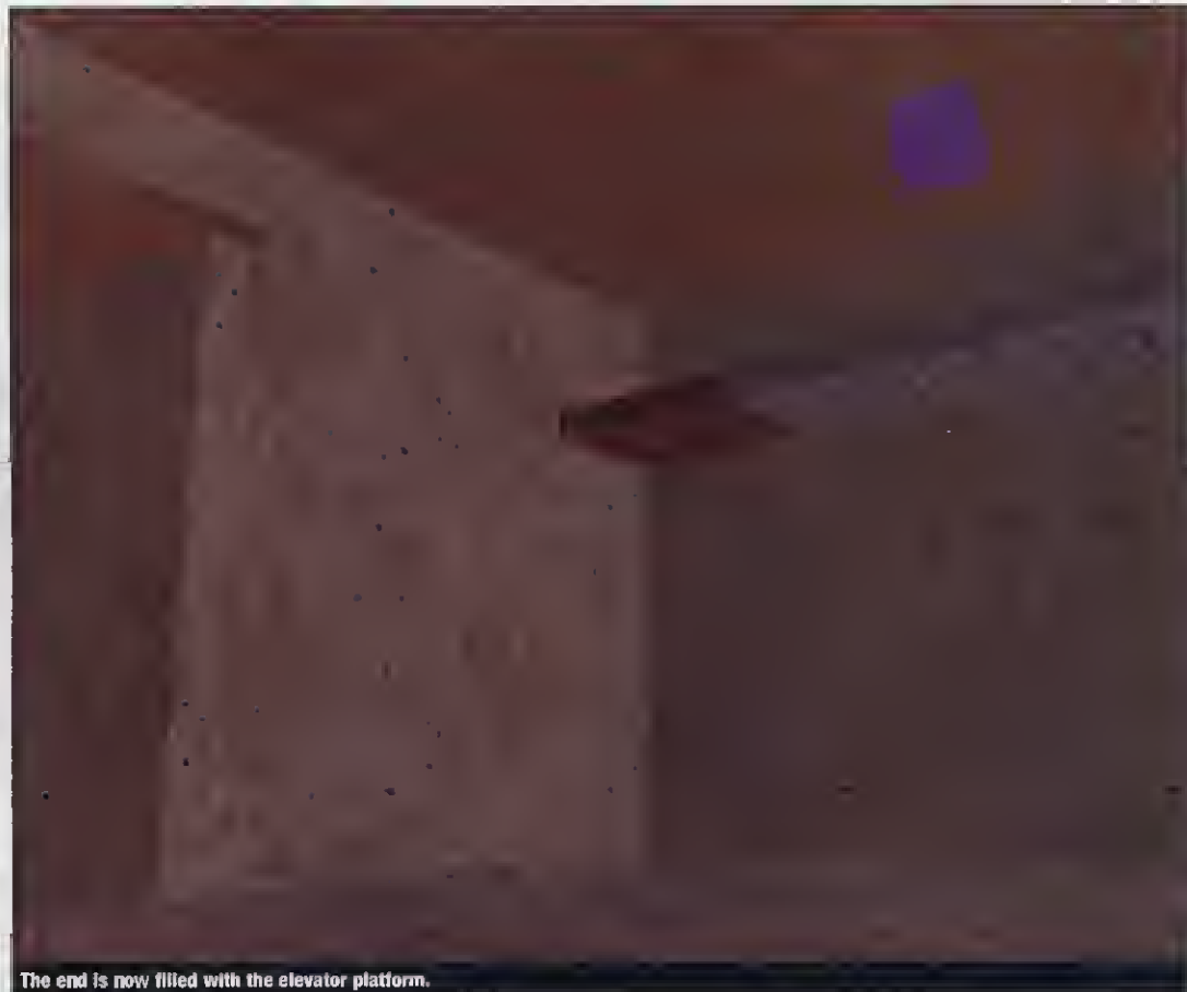
The end is now filled with the elevator platform.
